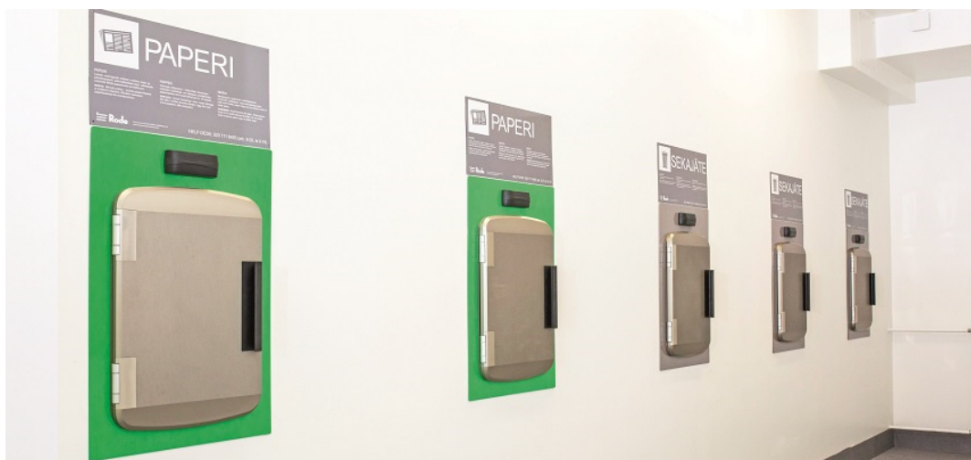
Waste hatches installed in the wall of a building.
