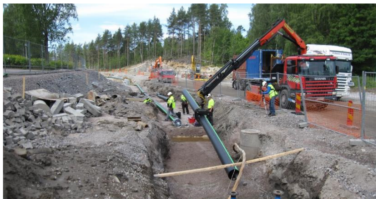
Approximately 10 kilometres of the composite pipeline is to be installed in the Kruunuvuorenranta area. Through the pipe network, different waste sorts travel to the waste containers located in the waste transfer terminal.
